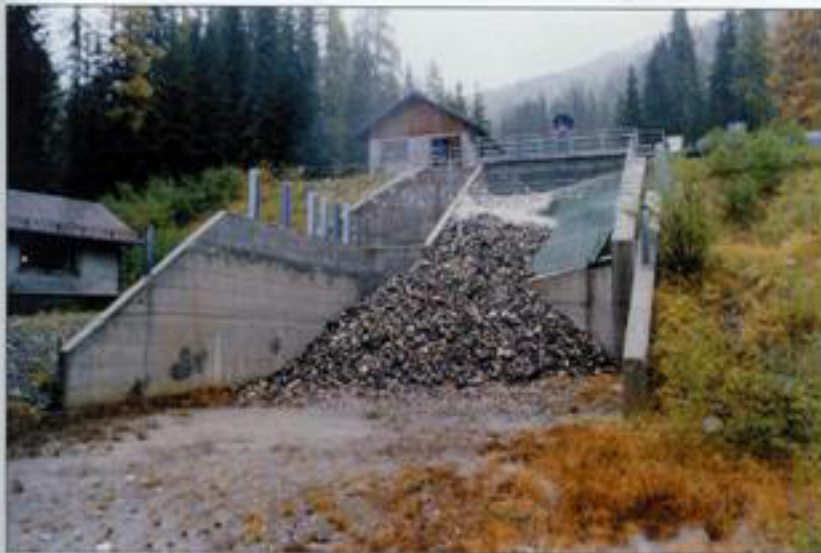
Photo 2 – The bedload deposited in the storage area after the October 1998 flood
