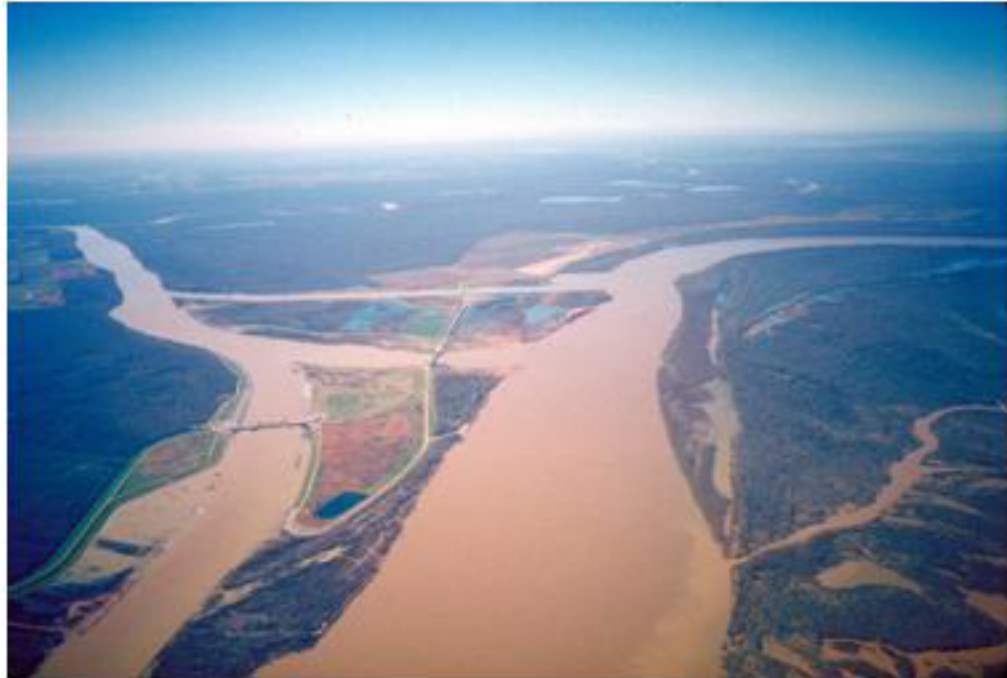
Old River Control Structure, Mississippi River
