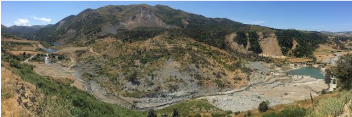
A large, long-lived landslide dam in North Canterbury formed during the 2016 Kaikōura-Hurunui earthquake
