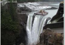
Figure 5. Removal of Glines Canyon Dam, Elwha River, WA.
